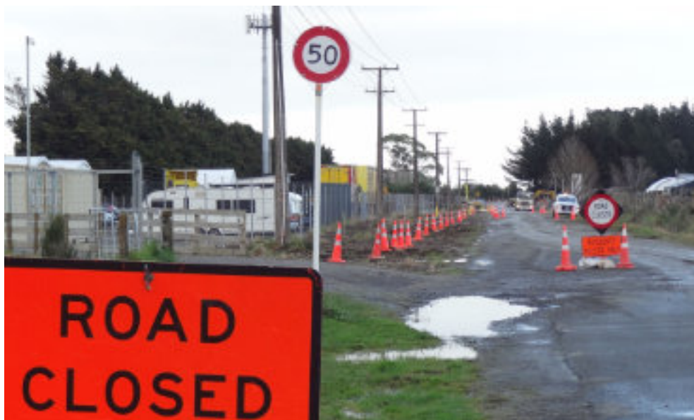
Photo: Road works begin on Custom Street
