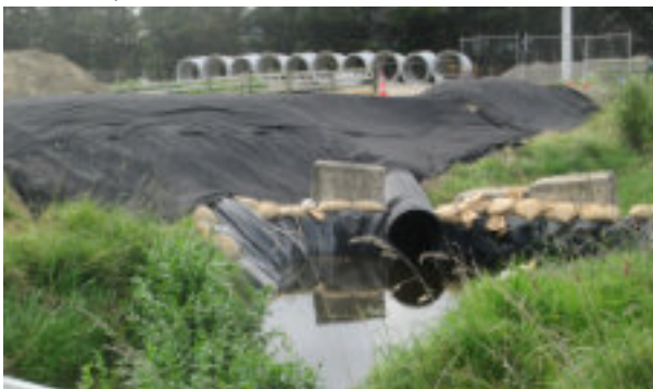
Photo: Pipes and stream diversion on Custom Street
