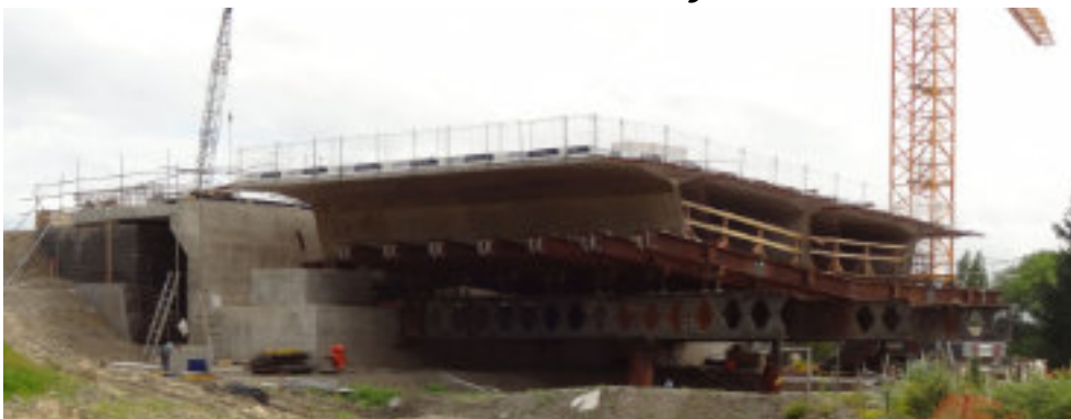
Photo: Construction progress of new bridge at Manawatū Gorge
