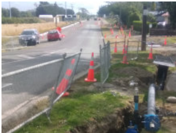
Photo: Ongoing road works in Custom Street
