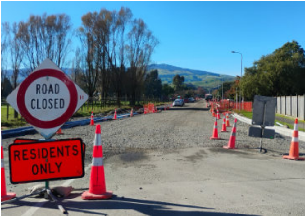
Photo: Wyndham Street Upgrades
