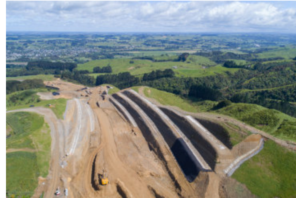
Photo: Cut 13 looking west towards Ashhurst.
