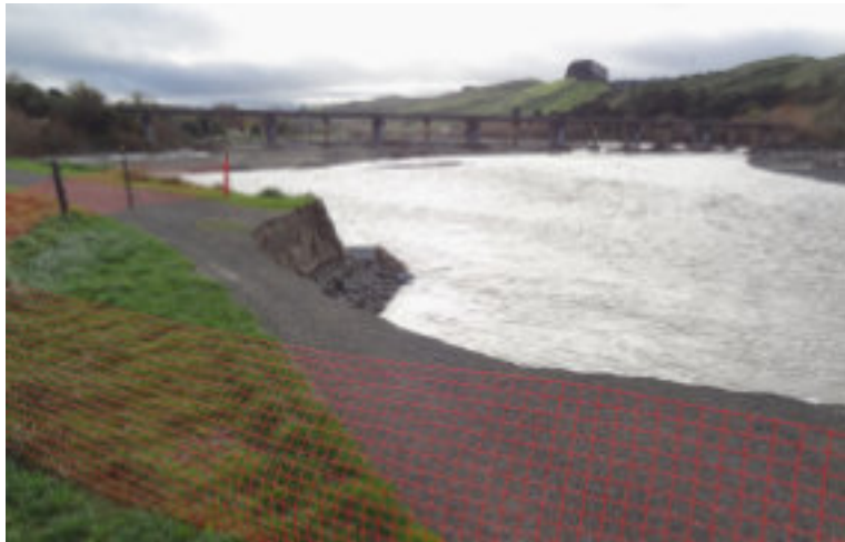
Photo: Domain path erodes near railway bridge
