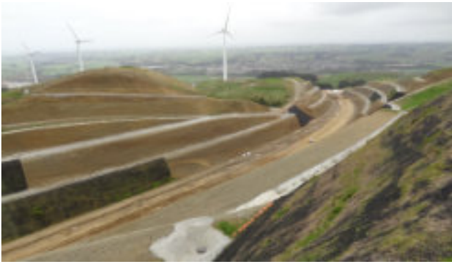
Photo: Te Ahu a Turanga cutting to Ashhurst
