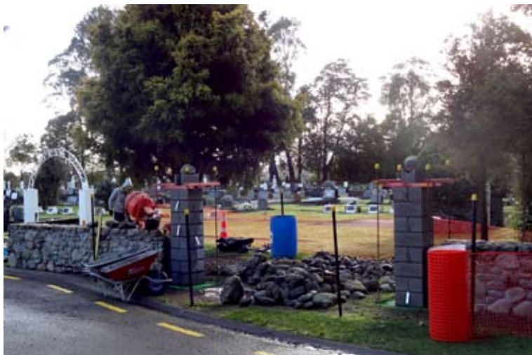
Photo: Construction of rock gateway at Ashhurst cemetery
